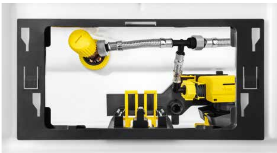
Shower WC connection in seconds: The adapter makes it possible.
